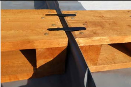
Detail of anchorage of a wooden ramp
