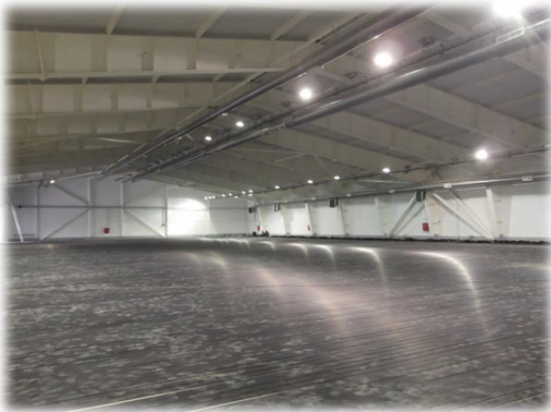
Krasnoyarsk, indoor heat insulation of the rink
