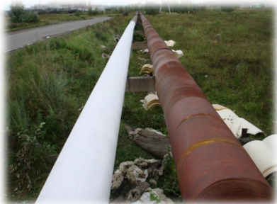
Krasnoyarsk, "Krasmath" - heat insulation of heat transport system
