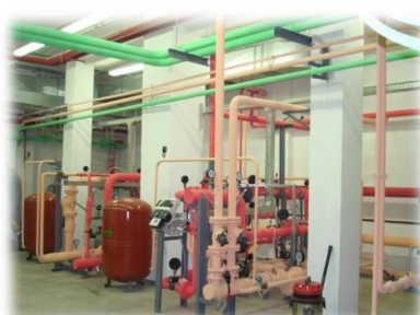
Krasnoyarsk, "Europe" Business Centre - heat insulation of pipelines
