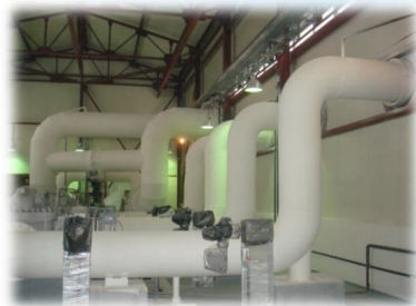
Krasnoyarsk Severnyy PNS - heat insulation of pipelines and equipment
