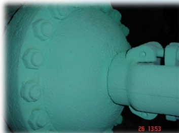
Krasnoyarsk, Electric Carriage Repair Plant - heat insulation of pipelines and equipment
