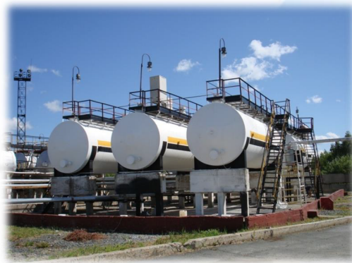
Achinsk, "ROSNEFT" Heat insulation of petroleum storage containers
