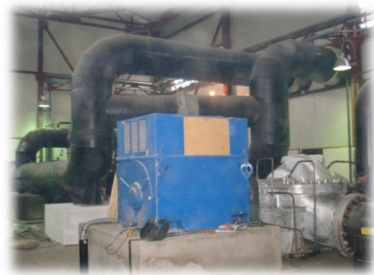
Krasnoyarsk, "Krasmath" - heat insulation of heat transport system
